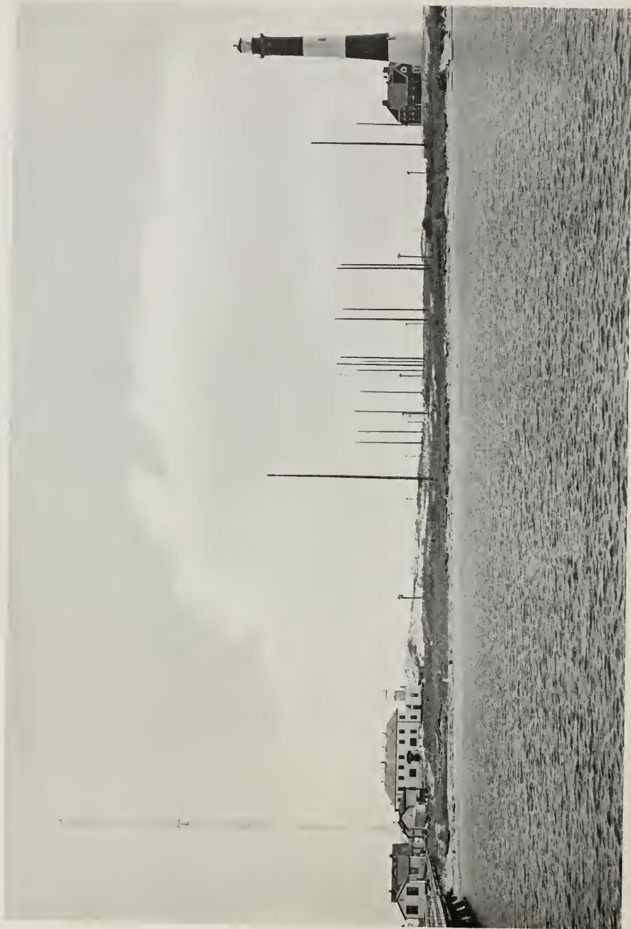
THE HIGH TOWER AND LOW MASTS AT THE U. S. COAST GUARD STATION ON FIRE ISLAND, N. Y., WILL BE USED IN CONJUNCTION WITH AN RCA HIGH-POWERED TRANSMITTER RECENTLY INSTALLED IN THE BUILDING AT THE LEFT.
